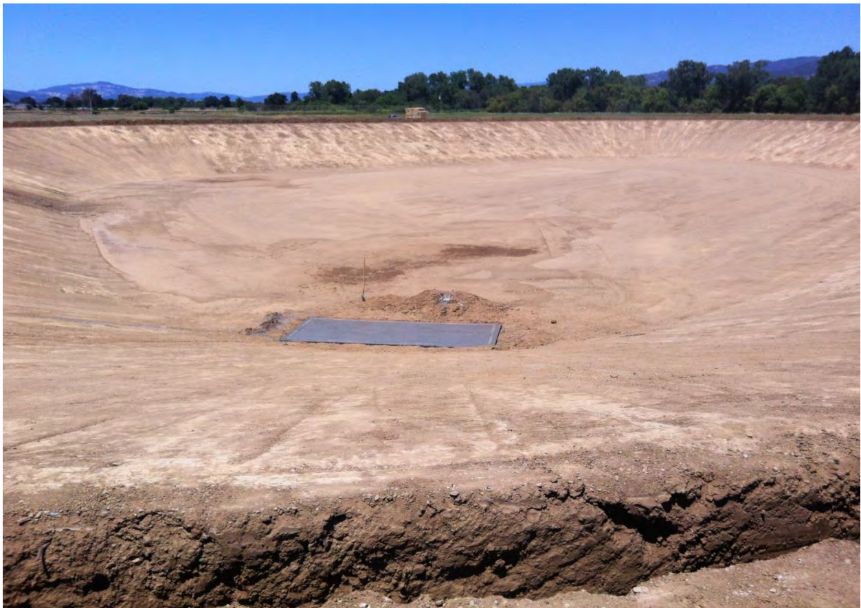
Figure 163. Offstream pond before and during grading
